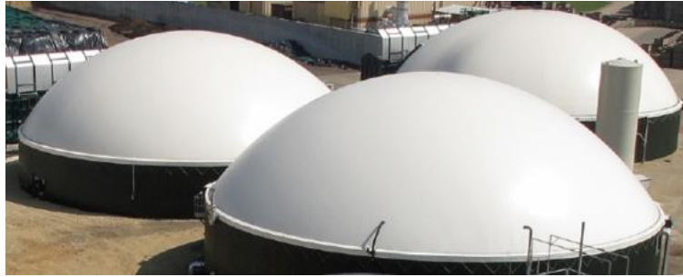
Figure 7 – wet anaerobic digestion tanks
