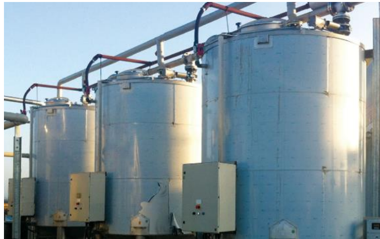
Figure 9 – Pasteurisers treating food waste following digestion
